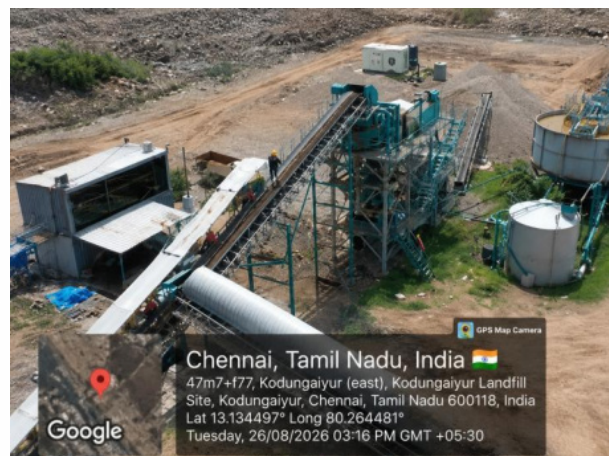
Aerial view of the Kodungaiyur (KDG) processing facility
