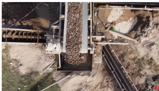
Screening and recovery of recycled aggregate from C&D waste
