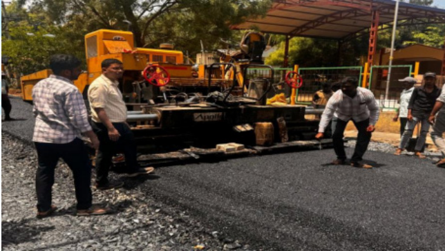
Laying the plastic-modified bituminous mix on the prepared road surface
