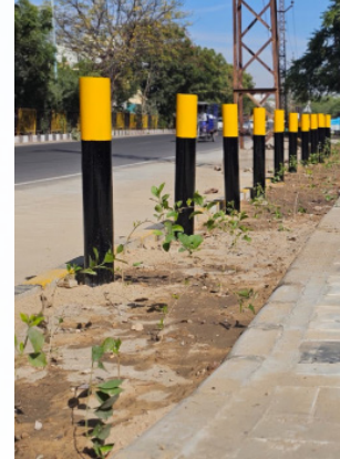
After — completed interlocking-block footpath
