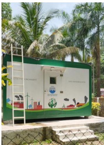
Station cabin sited amid a coastal industrial belt
