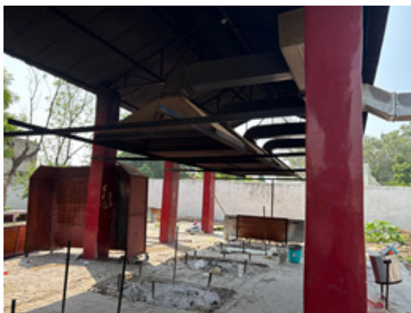
After — completed smoke-capture hoods and ducting network
