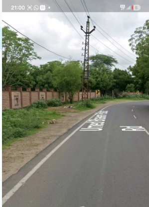
Before — unpaved, dust-generating roadside shoulder
