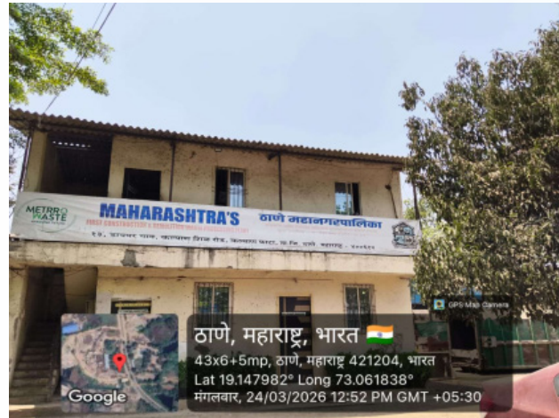
Facility building — “Maharashtra’s First Construction & Demolition Waste Processing Plant”
