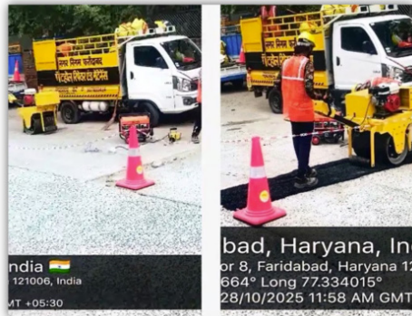
Pothole Repair & Maintenance van and equipment deployed on site, Sector 8, Faridabad
