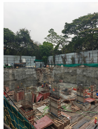
A monitored construction site (excavation and foundation stage) within PMC limits
