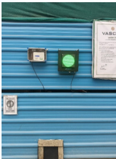
Green LED indicator and sensor at a site gate
