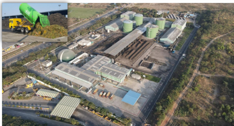
Aerial view of Indore Municipal Corporation's 550 TPD Gobardhan Bio-CNG Plant.
