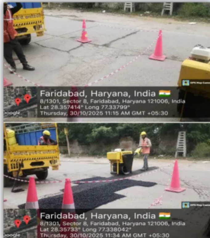
Pothole repaired — bituminous patch laid and compacted, Sector 8
