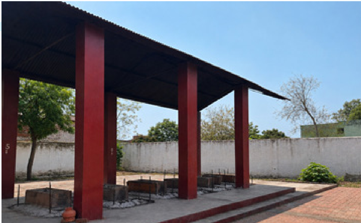
Before — open pyres at the crematorium, without emission capture
