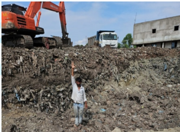
Before — garbage dumping yard under clearance and site preparation
