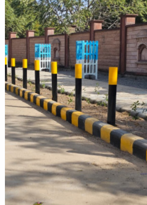
After — paved footpath with kerb separation and protective bollards
