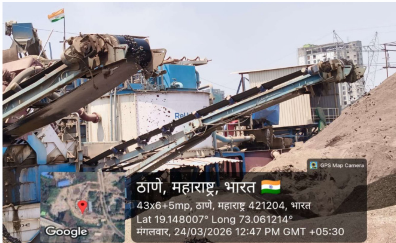
Crusher and conveyor system processing C&D waste at the facility
